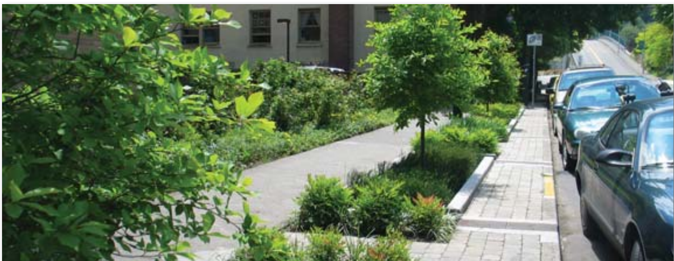
STREETSCAPE UTILIZES GREEN INFRASTRUCTURE PRACTICES (BIORETENTION AND POROUS PAVEMENTS) TO REDUCE AND IMPROVE THE QUALITY OF STORMWATER RUNOFF - PROTECTING NATURAL RESOURCES.
