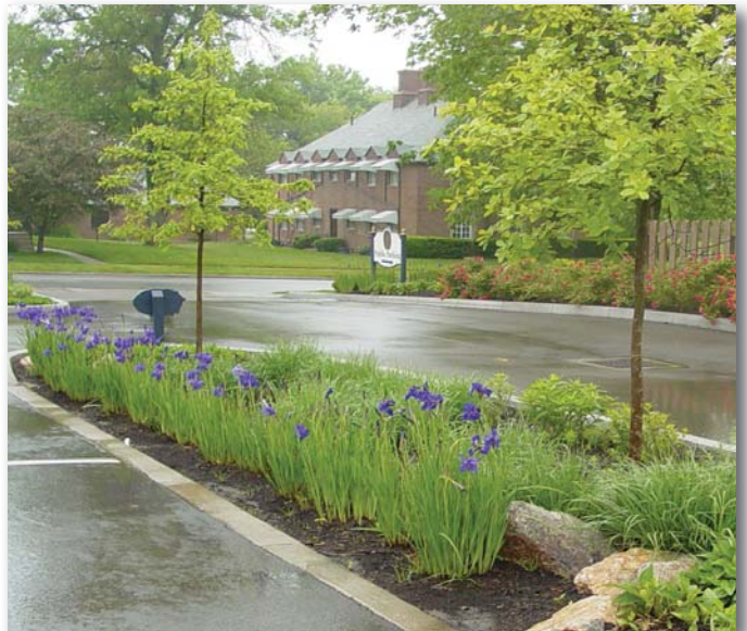
DEPRESSED TREE ISLAND IN PARKING LOT
