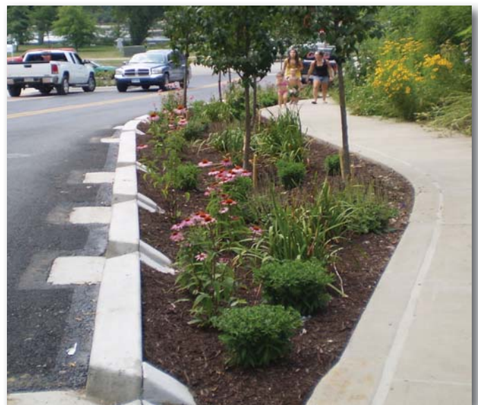
STORMWATER DIRECTED TO BIORETENTION AREAS
